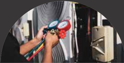
Air Conditioning Equipment
