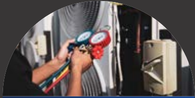
Air Conditioning Equipment
